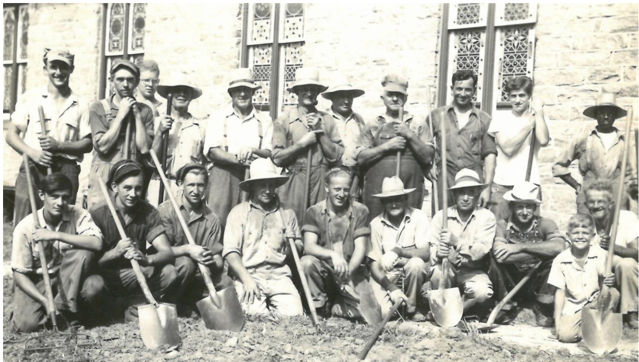
The work crew that created the basement to the church sanctuary, 1945 (Young Tom Swift is kneeling in the lower right)
